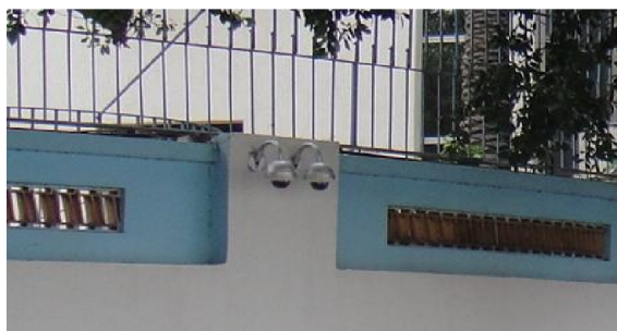
FIG.26 – Typical installation of CCTV external camera
